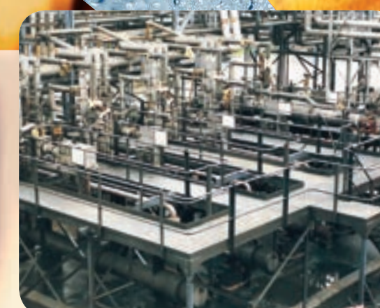
Heating cracked-bottoms and coal tar mixture Heating to 280°C+: 28 years operation, negligible fouling. Previous plain tubes fouled to shut-down every 2/3 months
