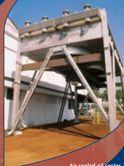
Air cooled oil cooler, Yibal. Client: Petroleum Developments Oman Courtesy: GEA, India
