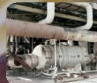
Paraxylene Feed Vapouriser/Reactor Effluent Interchanger. Increased duty to overcome capacity and space limitation. Courtesy: Huntsman Chemicals (ICI UK)
