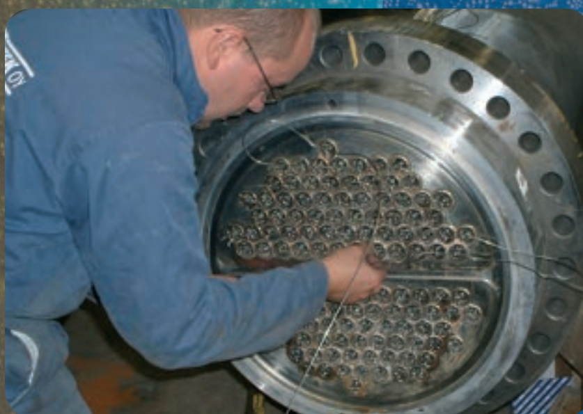
hiTRAN installation. Courtesy: KCC
