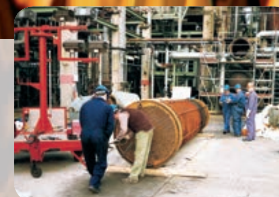
Hyssomer feed/effluent exchanger Correction of vapour flow maldistribution
